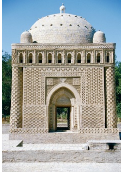
The Samanid dynastic tomb in Bukhara, tenth century. The Samanids were known for their fine decorative brickwork, and the tomb exhibits their skill on both the exterior and interior walls.
